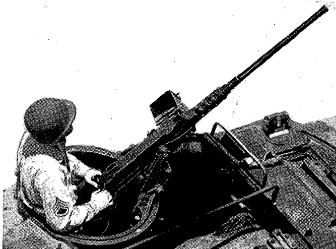
FIGURE 30.—Concentric ring mount.
