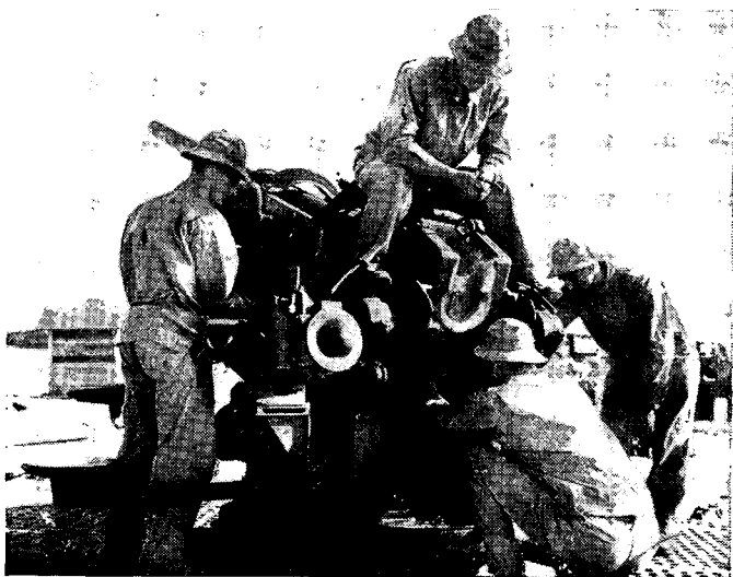
© Pushing out spline shaft. (Note position of breechblock support.)
