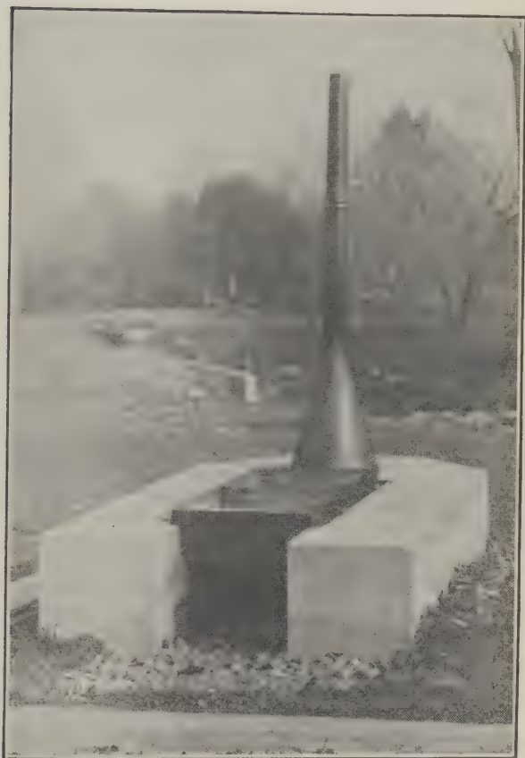
FIGURE 26.—Guthrie drying pan incinerator.
