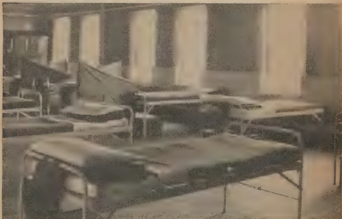
FIGURE 2.—Method of constructing cubicles in squad rooms by the use of shelter tent halves with head and foot arrangement of beds
