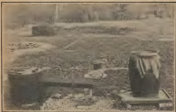
FIGURE 30.—Soakage pit and grease traps. Left, cold water grease trap; right, ash barrel grease trap.
