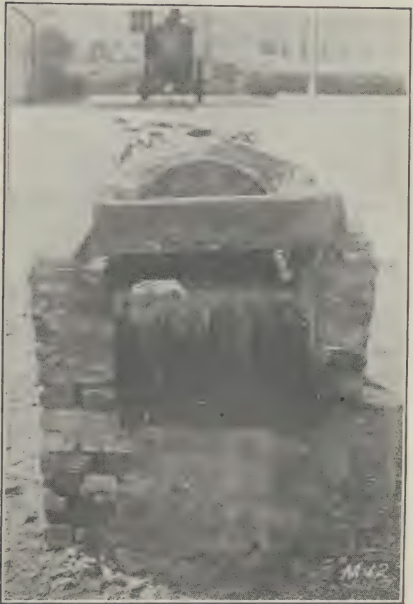
FIGURE 19.—Incline plane incinerator, end view.
