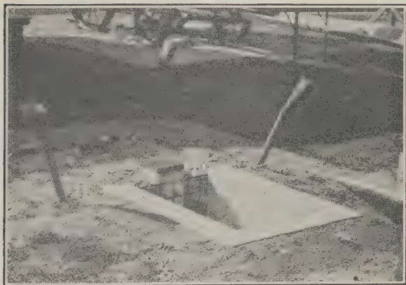
FIGURE 13.—Urine soakage pit.
