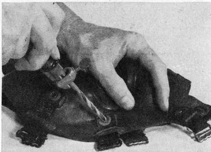
FIGURE 74.—Shank being reamed out with reaming tool.
