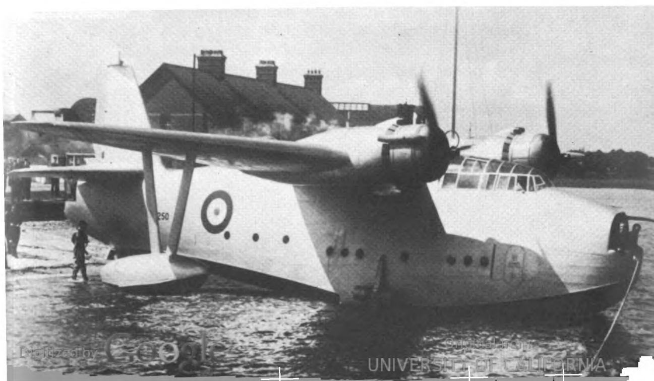
Britain's newest long-distance flying boat is the Saro Lerwick. This picture shows the original prototype being launched for the first time. It has a wing span of 81 feet, a length of 63 feet, and a height of 20 feet. Engines are 1,100/1,150-h.p. Bristol Hercules.
